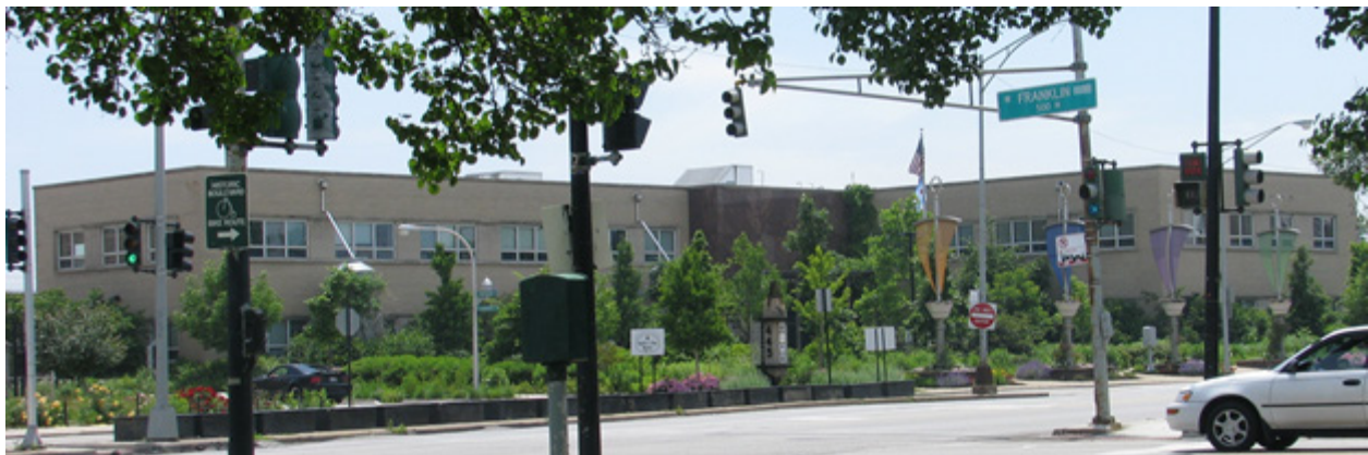
Figure 20.1. Chicago Center for Green Technology (Source: Chris DeSousa, June 2009).
