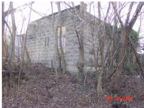
Front of Building. Source: U.S. EPA OSC. 2008
