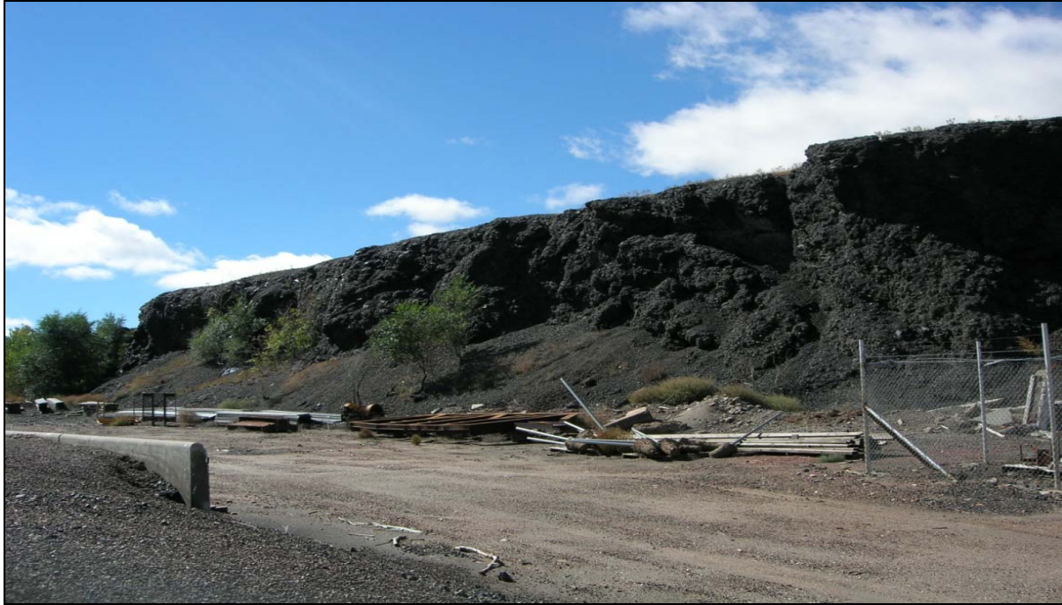
Figure 2. Slag pile and broken perimeter fence, Colorado Smelter site, Pueblo, Colorado
